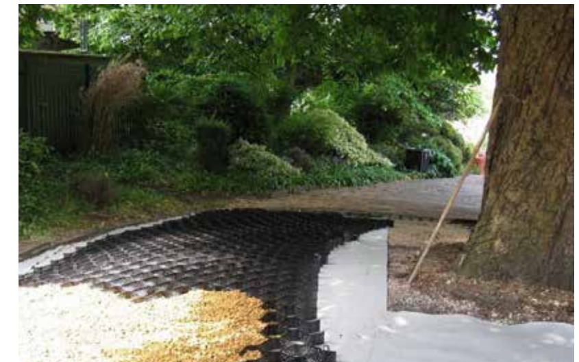
No-dig construction of footpaths allows routes within tree RPAs, creating scenic and varied routes through the wooded landscape
