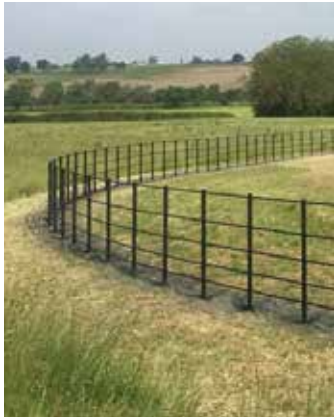
Steel estate railings
