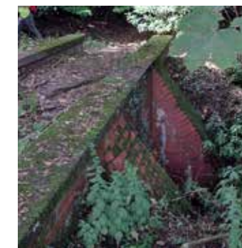
07 Footbridge over culvert
