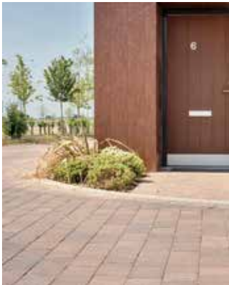
Carriageway and footways - Tumbled concrete block paving, Traditional colour
