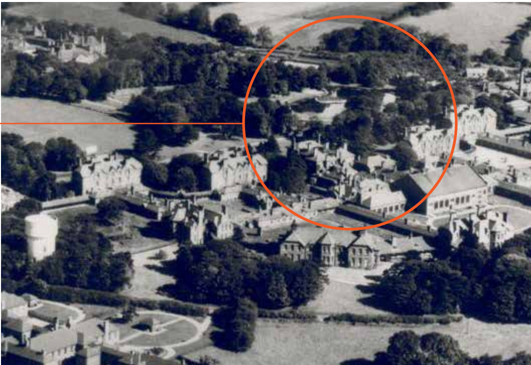
Historical photo of site (Source: www.whittinghamhospital.co.uk )
